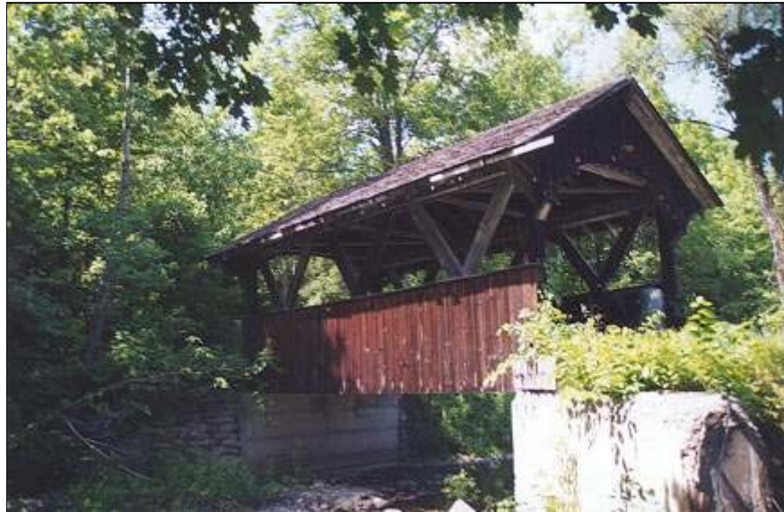
Photo of Waldbillig Bridge
