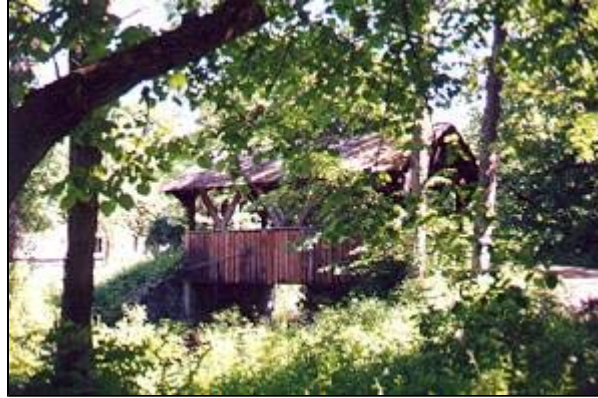
Photo of Waldbillig Bridge
