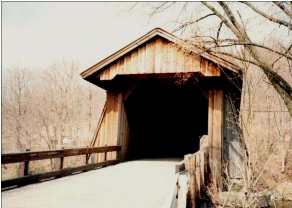
Van Tran Flat Bridge Portal
