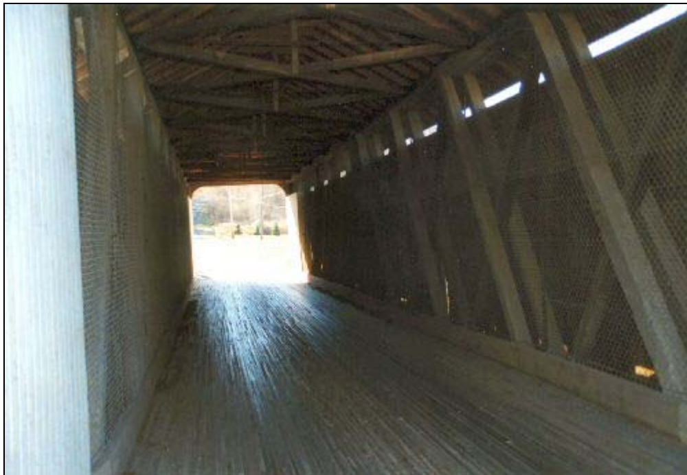
Rexleigh Bridge Truss
