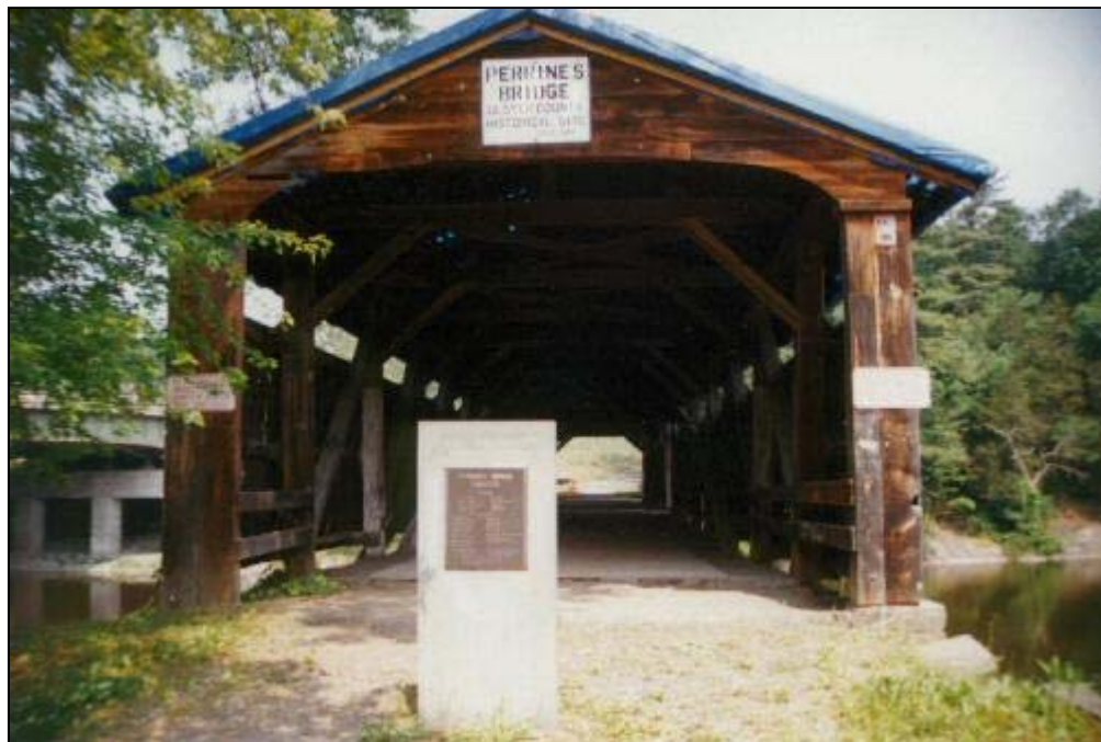
Perrine's Bridge Portal
