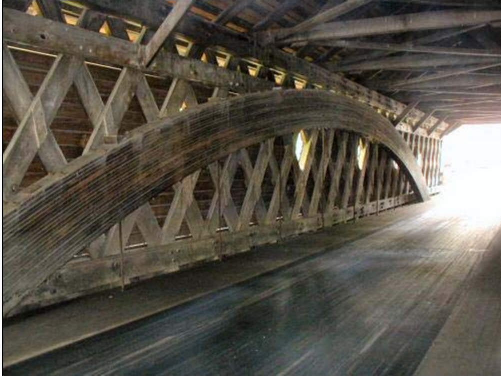
Town Lattice Truss and Arch
