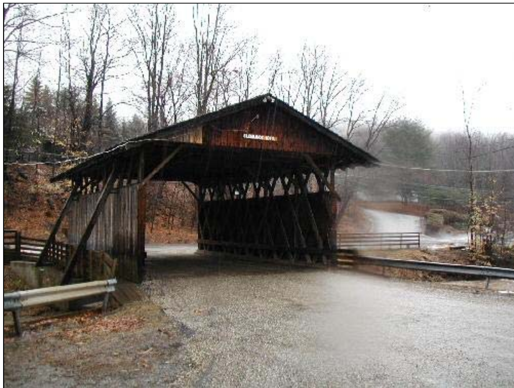
Photo of Grahamsville Bridge Portal during flooding in April 2005
