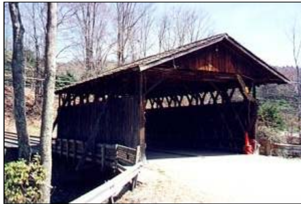
Photo of Grahamsville Bridge Portal
