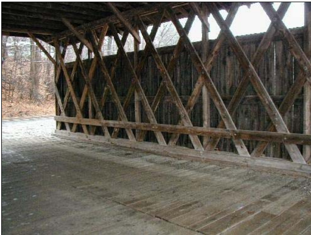
Photo of Grahamsville Bridge Truss
