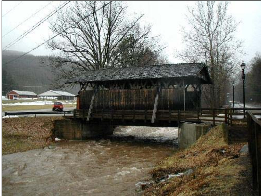
Photo of Grahamsville Bridge during flooding in April 2005
