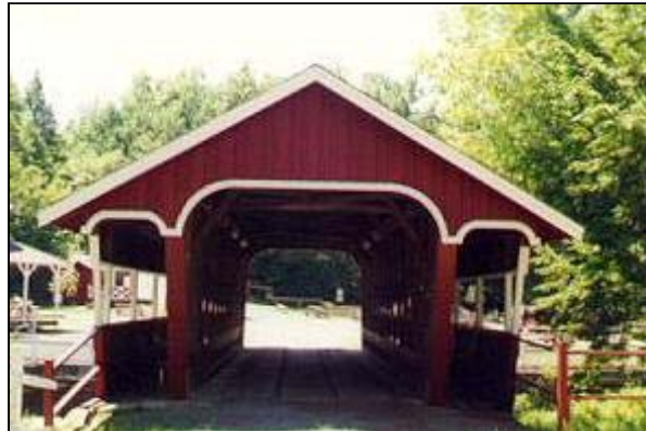
Eagle Mills Bridge Portal
