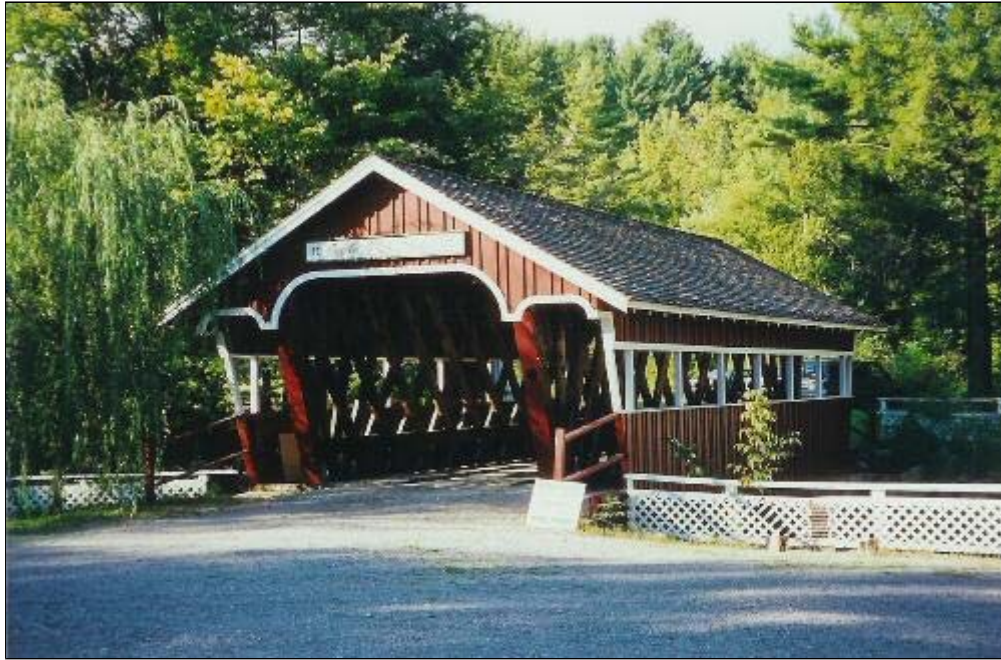
Photo of Eagle Mills Bridge
