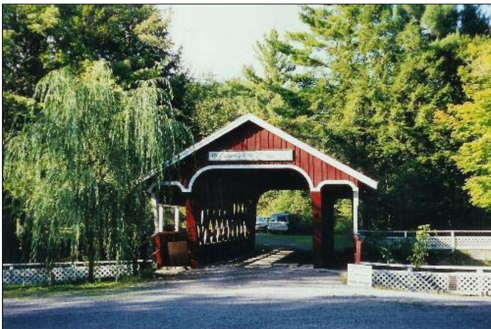
Eagle Mills Bridge Portal
