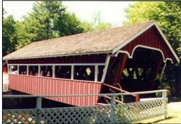
Photo of Eagle Mills Bridge
