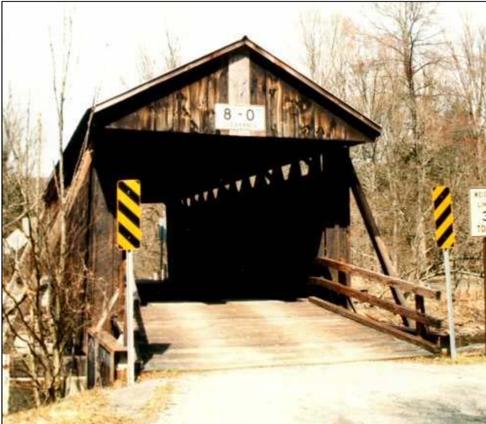
Bendo Bridge Portal
