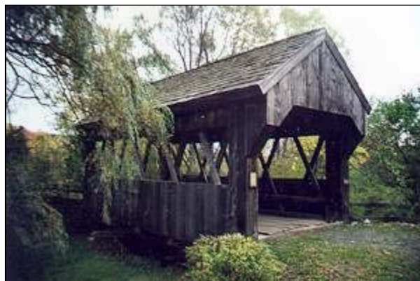
Photo of Americana Village Bridge
